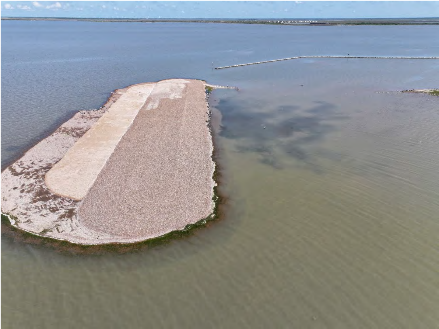
Rock reef restoration completed.
