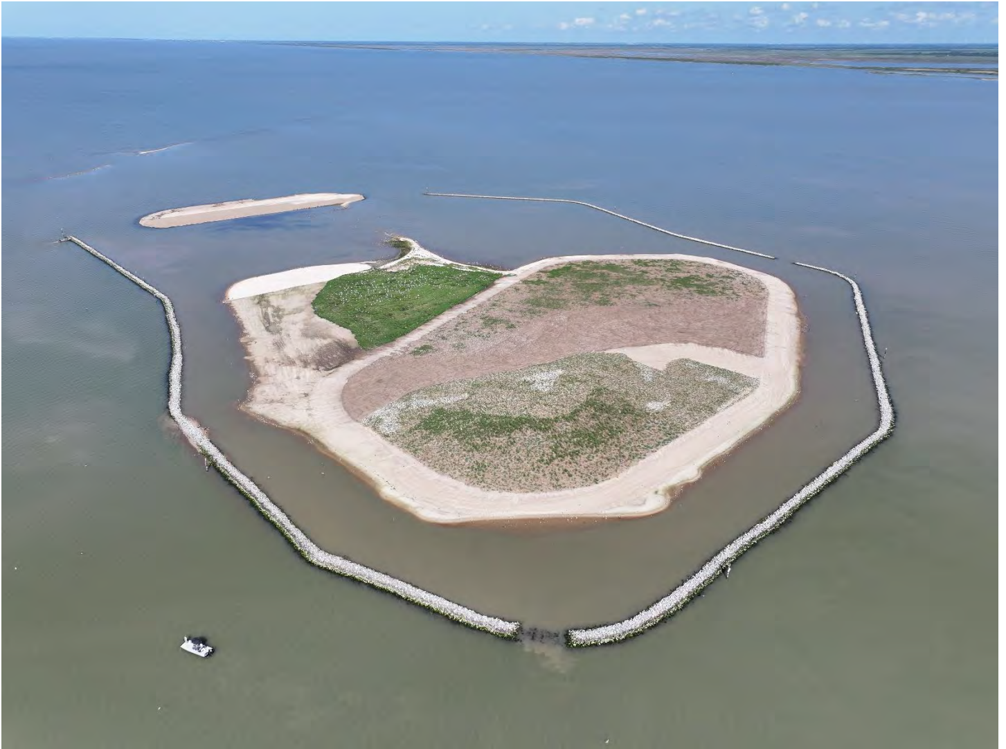
Dressing Point Phase 1 and 2 fully completed.
