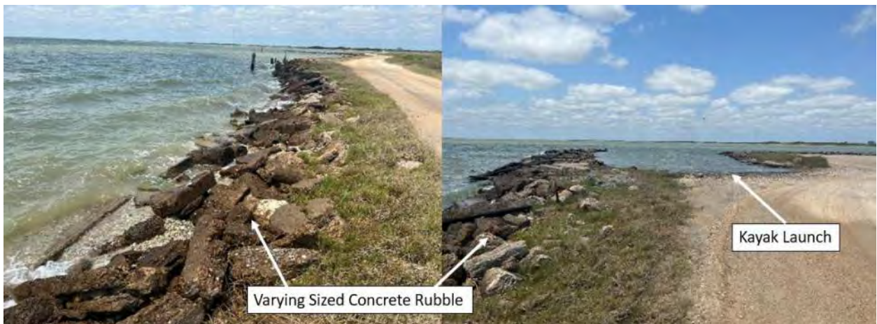
Figure 5 Concrete rubble revetment and kayak launch area.
