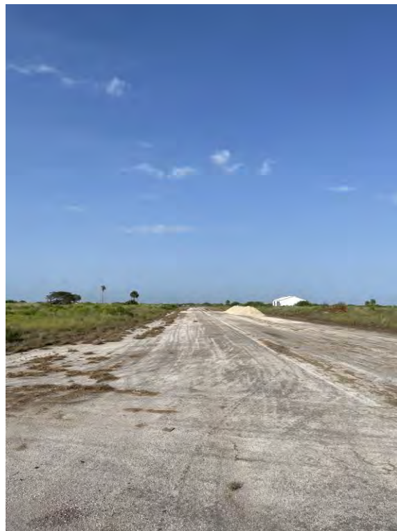
Photo 6. Base material on the southern runway brought in from the north (facing south).
