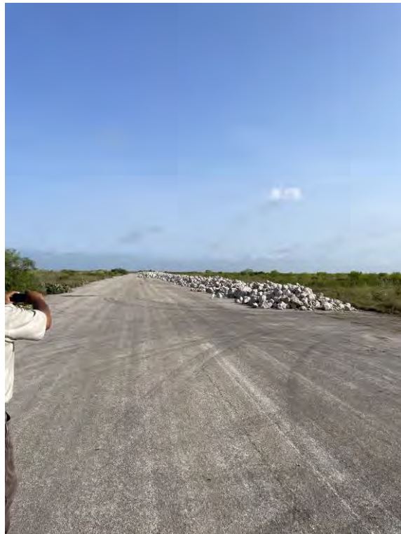
Photo 7. Stockpile of revetment stone on western part of runway (looking west).
