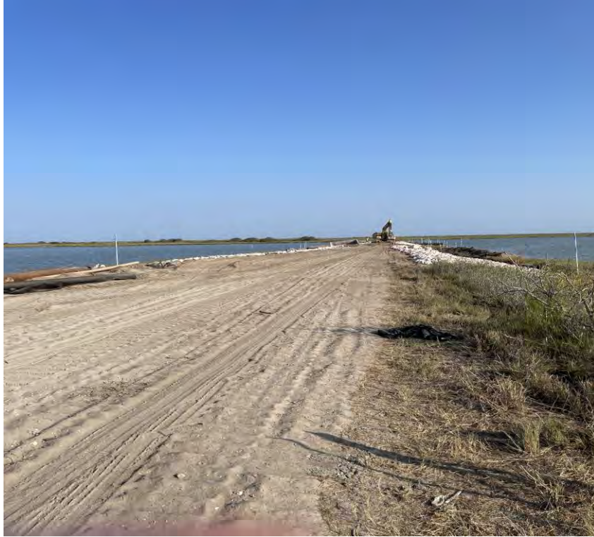
Photo 1. South end of B-SR-1 (looking north).
