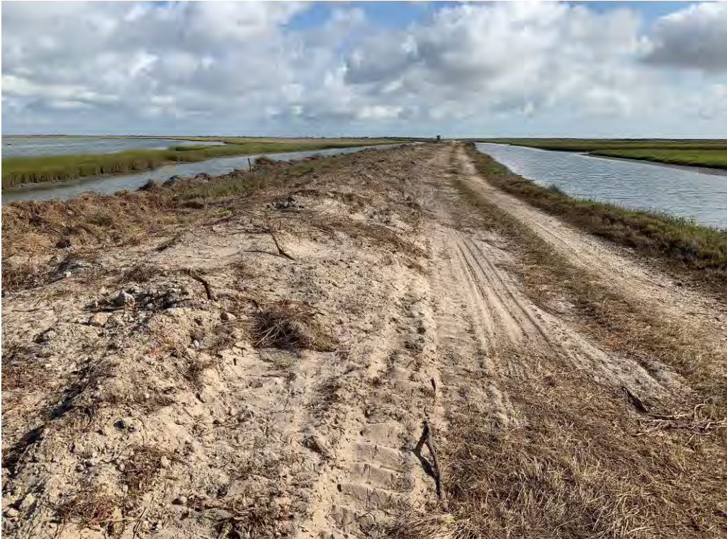
Photo 1. South end of cleared sand stockpile near B-SR-1 (looking north).
