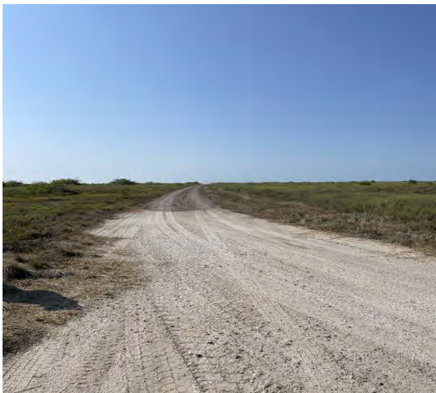
Photo 6. Repaired road that connects to FH-SR-3 at dried watering hole (facing south)
