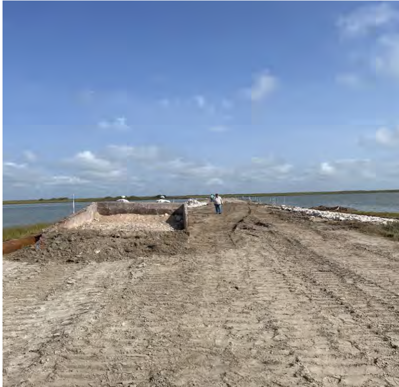
Photo 1. South end of B-SR-1 (looking north)
