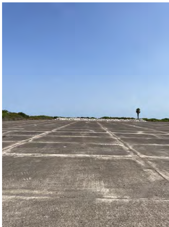
Photo 8. Stockpile of revetment stone on north end of island to be transported.
