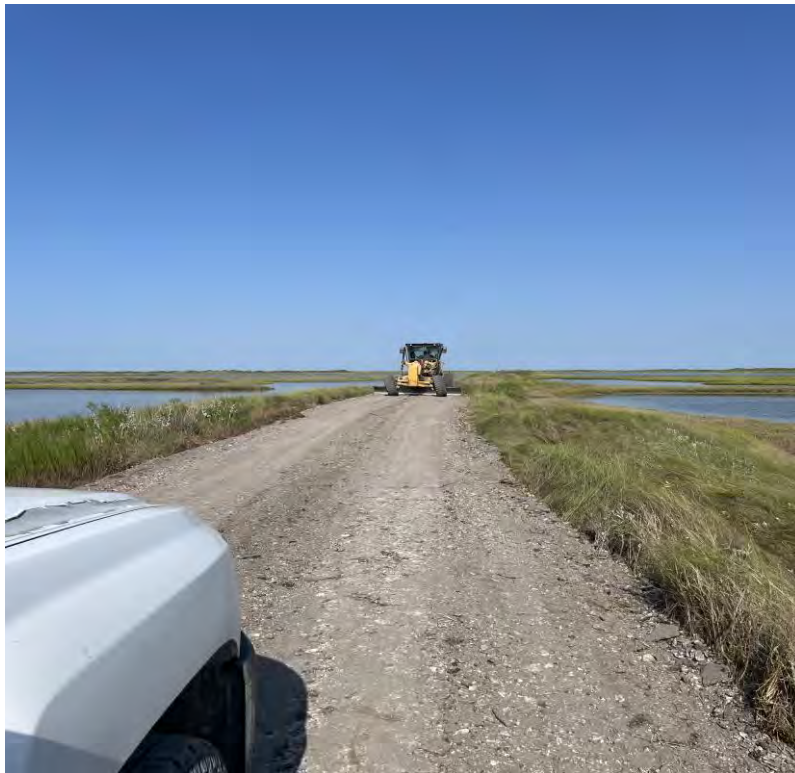
Photo 7. Grader constructing road towards FH-SR-3 site location (facing west)
