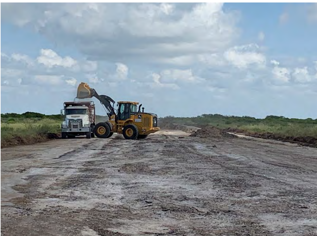
Photo 8. Loading reclaimed runway material into dump truck.
