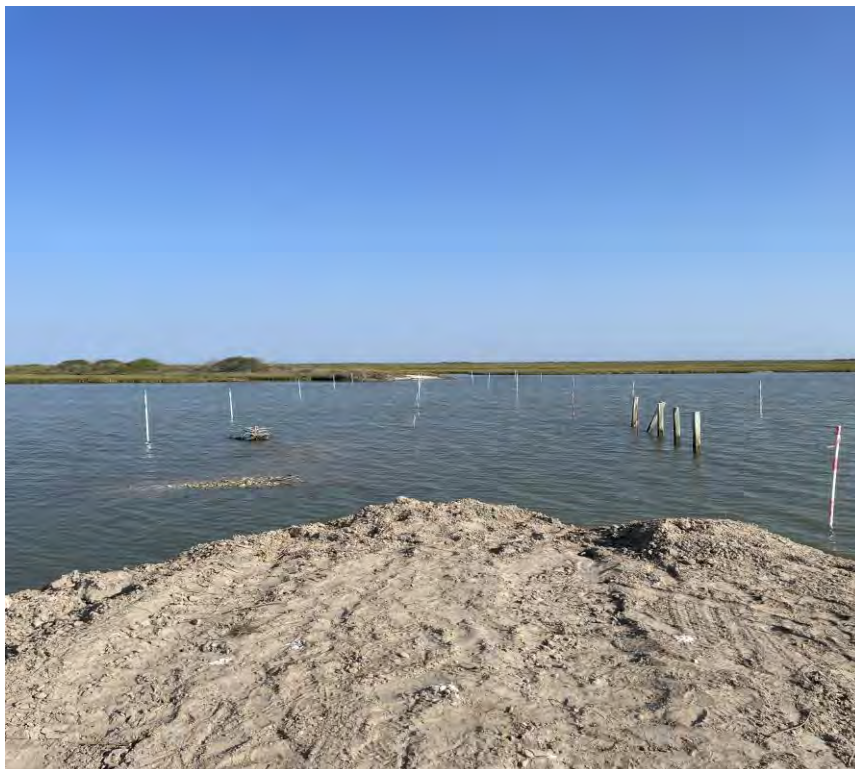
Photo 4. North extent of levee material placement (facing north)
