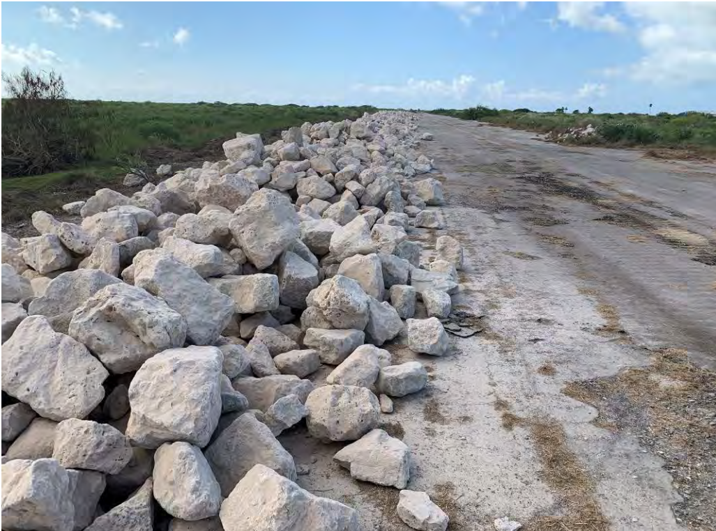
Photo 7. Stockpile of revetment stone on south runway (looking south).
