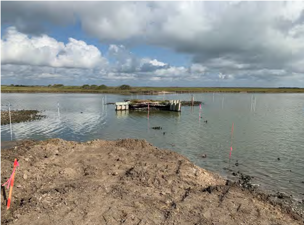
Photo 5. Area to be filled at B-SR-1 (looking north). Pink states denote levee roadway limits.
