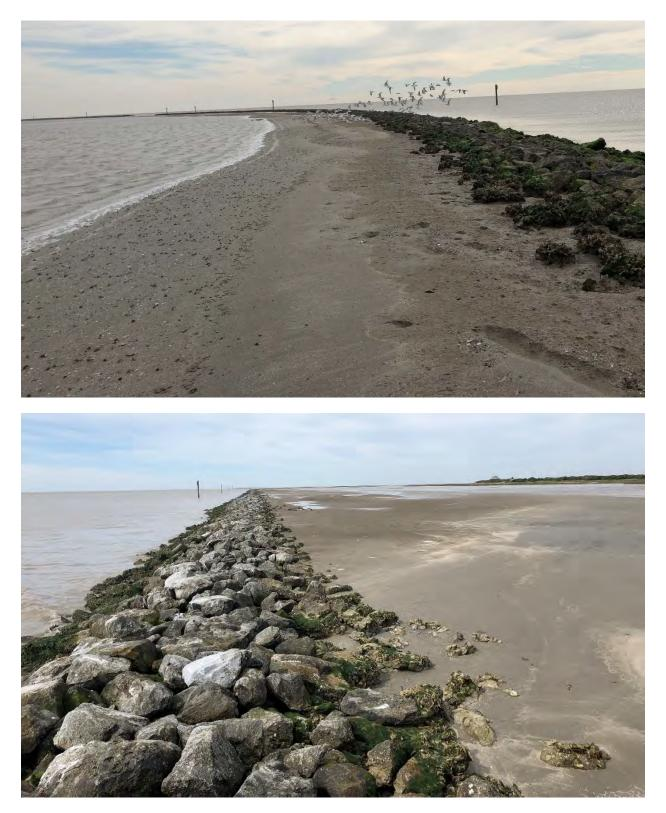
Figure 16. Sediment accumulation behind the Schicke Point living shoreline on March 5, 2019, 22 months post-construction.
