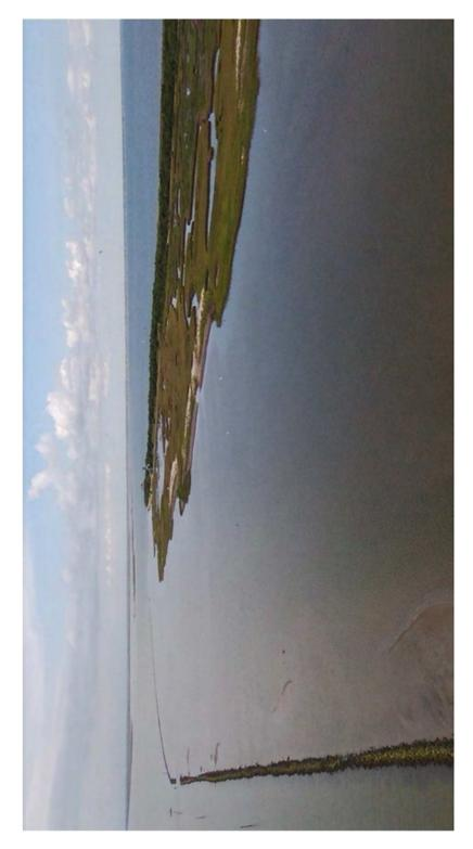
Figure 2. Schicke Point living shoreline constructed in May 2017 showing bands of sediment accumulation and Smooth Cordgrass/oyster marsh complex behind the living shoreline (July 6, 2018). Coastal forest visible in the background.
