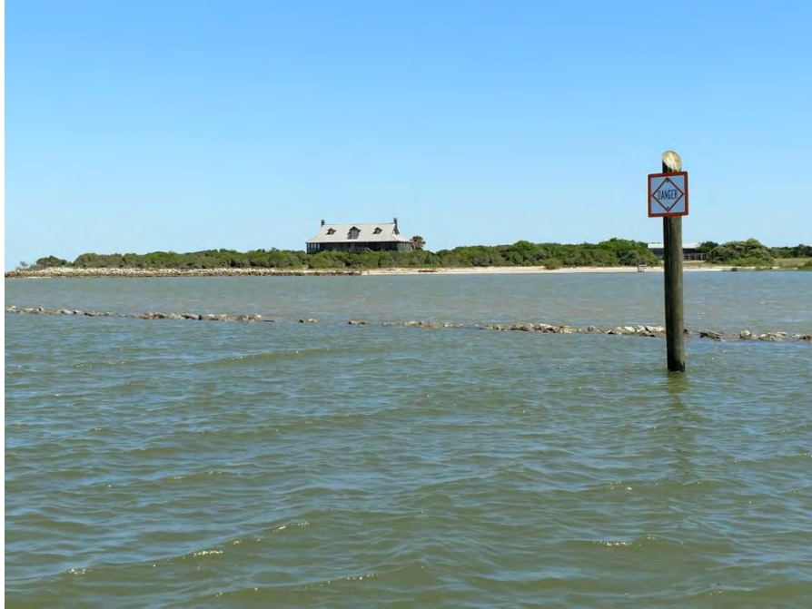
Figure 5. The photograph was taken from the Matagorda Bay facing north towards Schicke Point. The photograph shows the existing living shoreline at high tide. The new breakwater extension will be designed to be 1 foot above MSL (+1.74 NAVD88). The photograph was taken by Dave Buzan, FNI, in February 2020.
