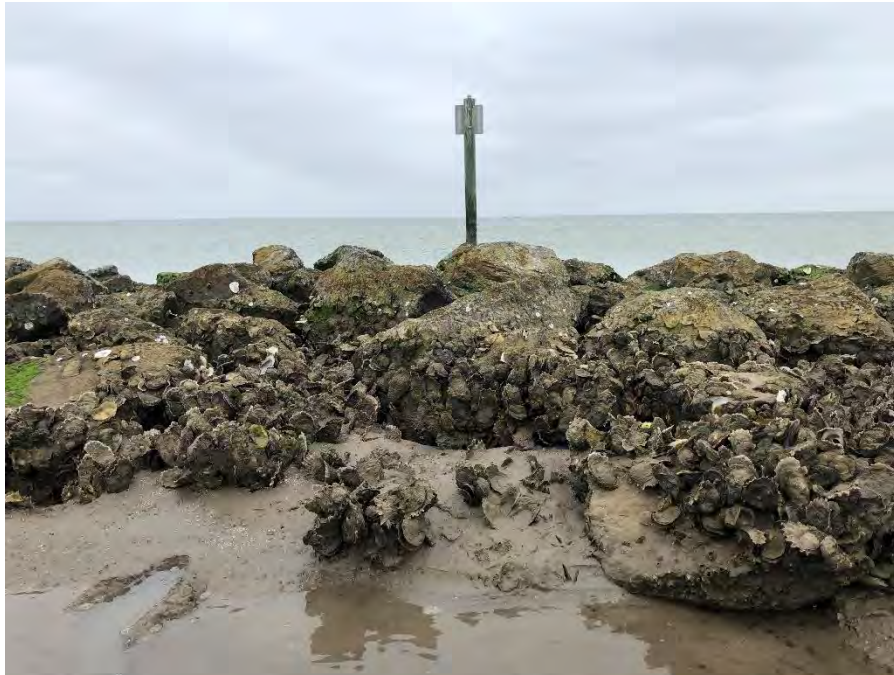
Figure 1. The photo was taken from the existing Schicke Point living shoreline from the shore side facing southeast towards the Matagorda Bay. The Schicke Point living shoreline was constructed in 2017. The photo shows the extent of oyster colonization along the rock riprap and sediment accumulation during low tide. The photograph was taken by David Buzan, FNI, in February 2020.
