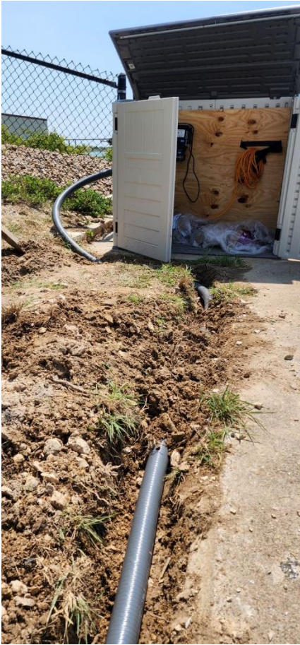
Figure 1. (Left) Trench running electrical extensions to grounded power outlet. (Right) Set-up and testing of electrical and water line connections.
